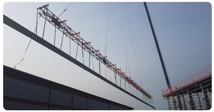
Look no further than the Modulift Lattice Spreader Beam! Said Melvyn Rogers at DSM Contract Lifting Service Ltd. "It is incredibly well built and very safe." The Modulift Lattice Spreader is designed for light loads that require multiple support points along its length.
